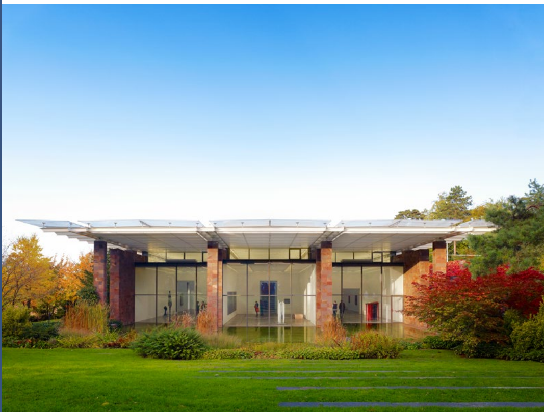
Fondation Beyeler, south facade, photo: Mark Niedermann
